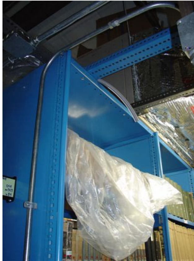
PLASTIC SHEETING IS A PERMANENT FIXTURE TO PREVENT WATER DAMAGE
