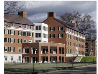
The new Fahey and McLane residence halls
