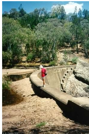
Koorawatha dams (early 1900s) : arch dams built for railway water supply (Australia). (Photos by Hubert Chanson, University of Queensland, Brisbane, Australia)
