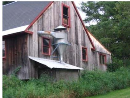
Cyclone separators have been used in the United States for about 100 years, and are still one of the most widely used of all industrial gas-cleaning devices. The main reasons for the wide-spread use of cyclones are that they are inexpensive to purchase, they have no moving parts, and they can be constructed to withstand harsh operating conditions.
