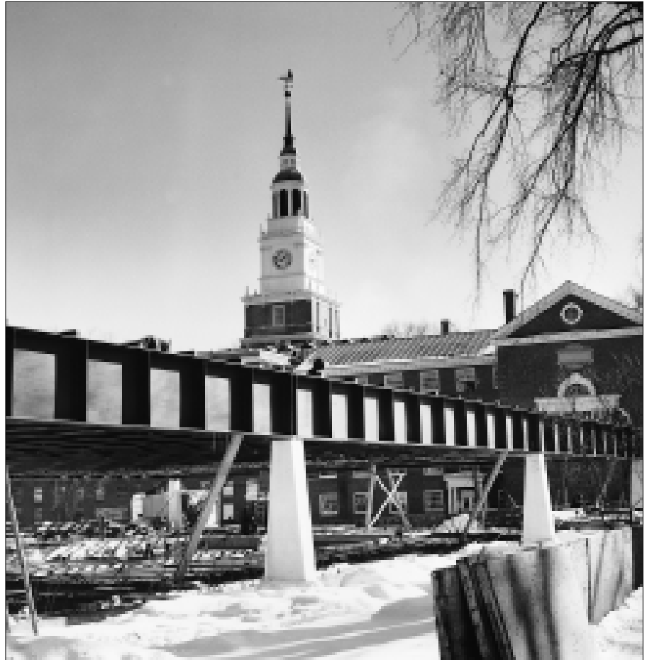
The Kiewit Computation Center under construction, 1965. (Archive photo)
