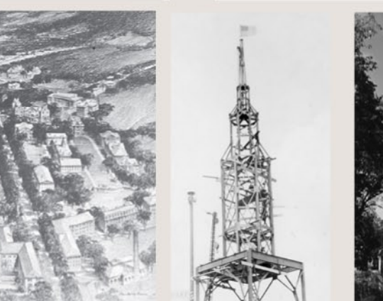
1927-8 Baker Tower construction and completion
